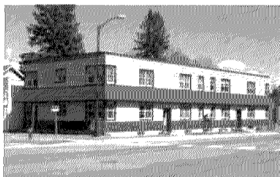
MRM Apartments (2013)- 105 NE 5 th St.
