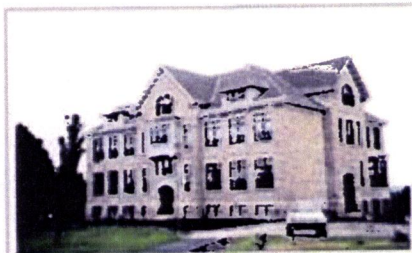
Mineral Point High School was converted to eleven apartments using historic preservation tax credits.
