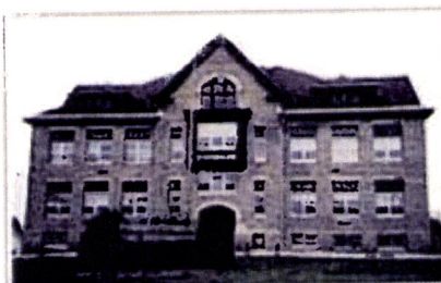
Mineral Point High School before restoration
