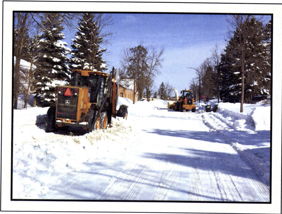
2013 Snow Plowing - Widening Roads and Improving Drainage
