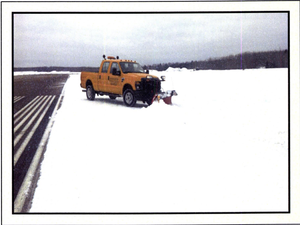
GR-Itasca County Airport – Clearing Off Lights on Runways
