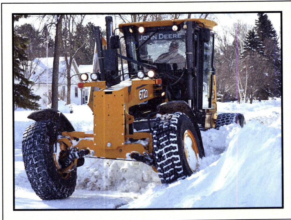
2013 Snow Plowing - Widening Roads and Improving Drainage
