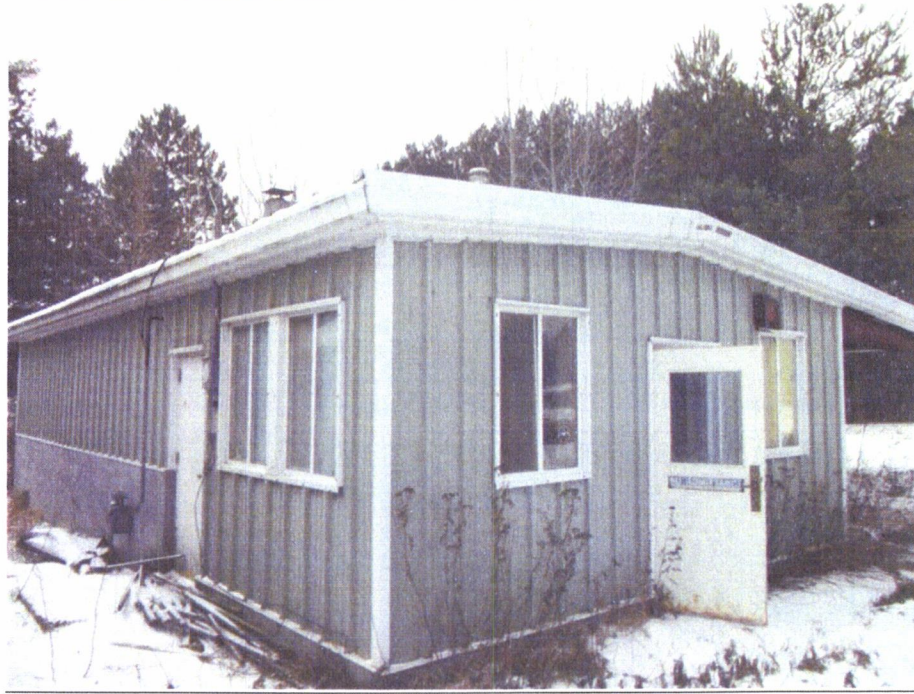
30' x 40' (1,360 sf) metal clad pole building (former dog pound)
