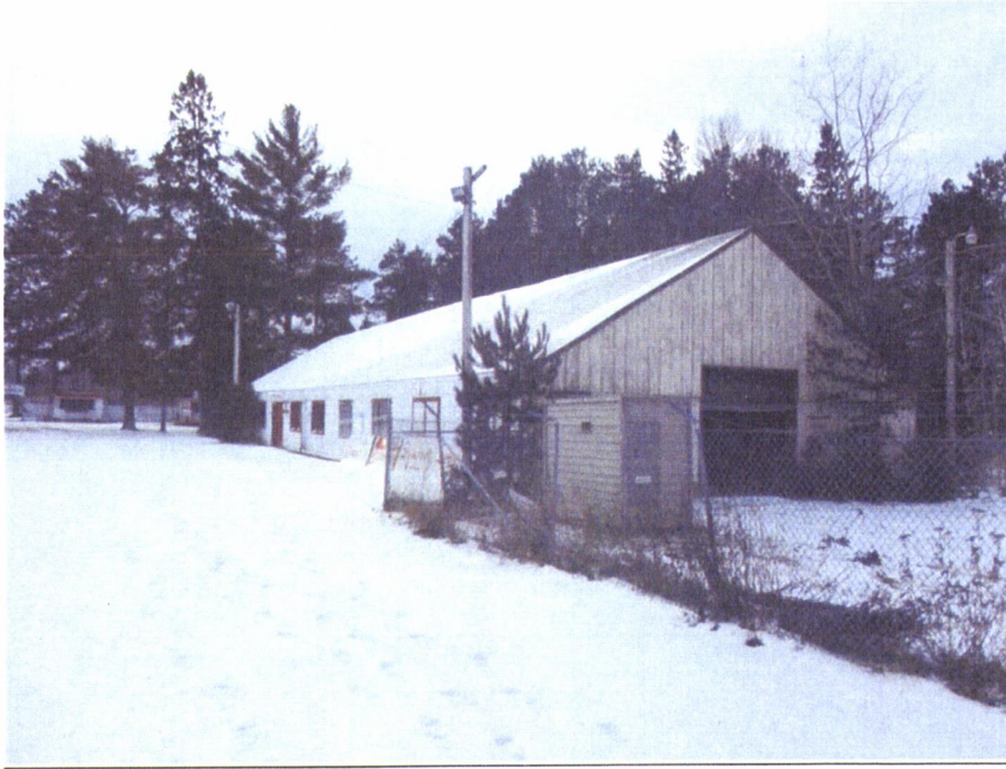
40' x 120' (4,800 sf) wood frame building
