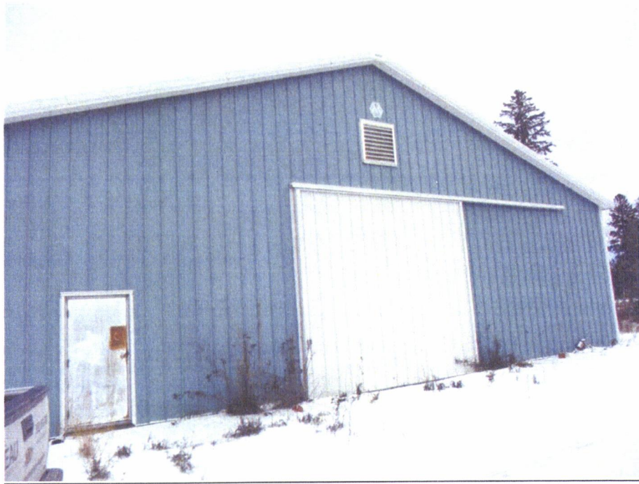
60' x 130' (7,800 sf) metal clad pole building (cold storage)
